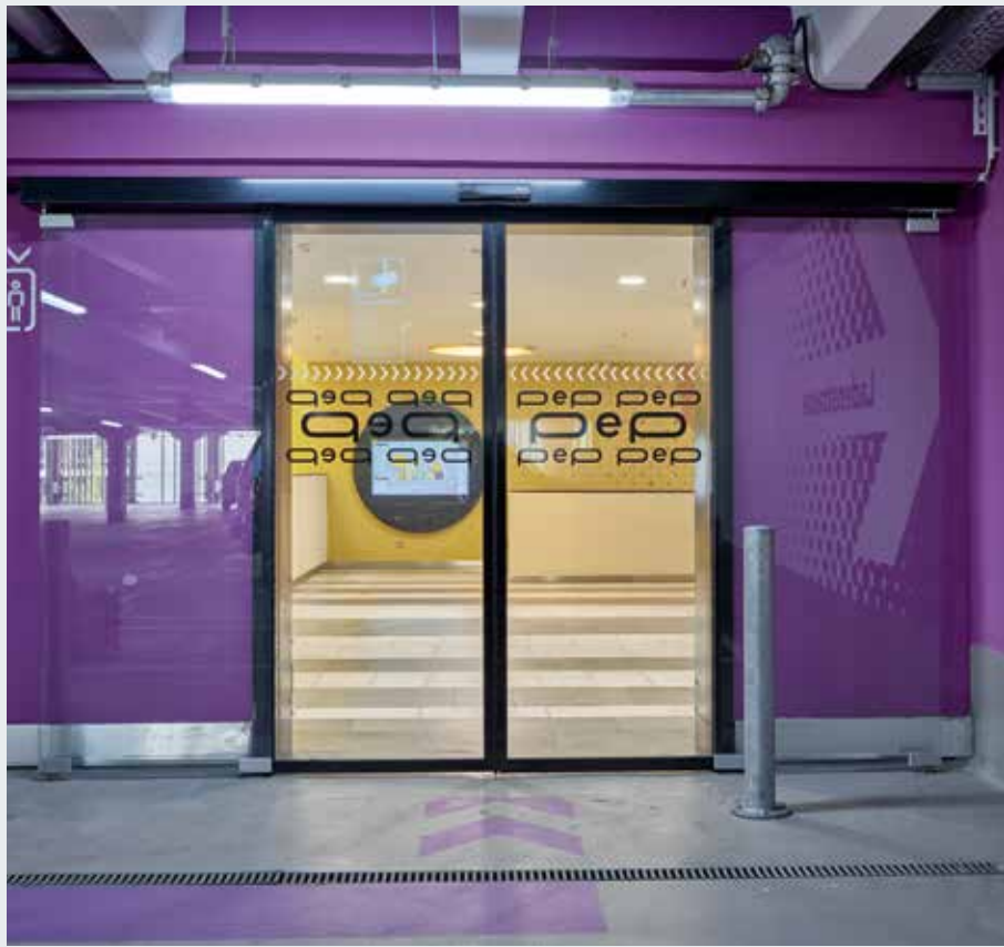
Viewed side of automatic sliding door
